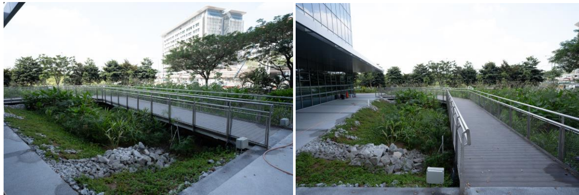
A walkway located above the rain garden to bring people closer to the feature
