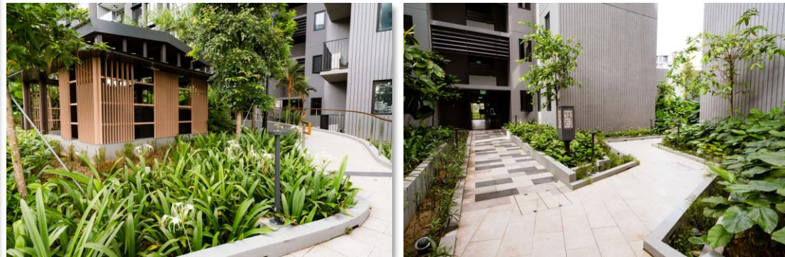
Rain gardens are well-dispersed throughout the residential blocks along the walkways
