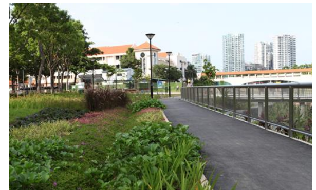
Bioretention Swale at Kallang River Potong Pasir
