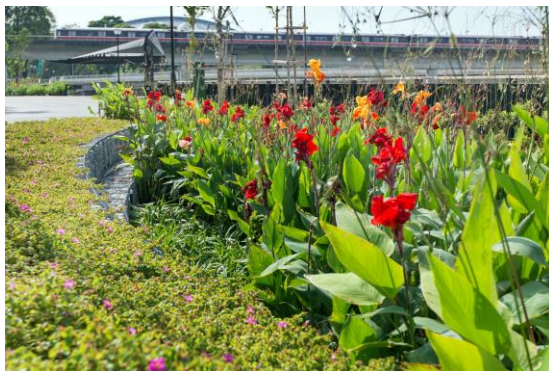
Rain Garden at Kallang MRT/BTOs
